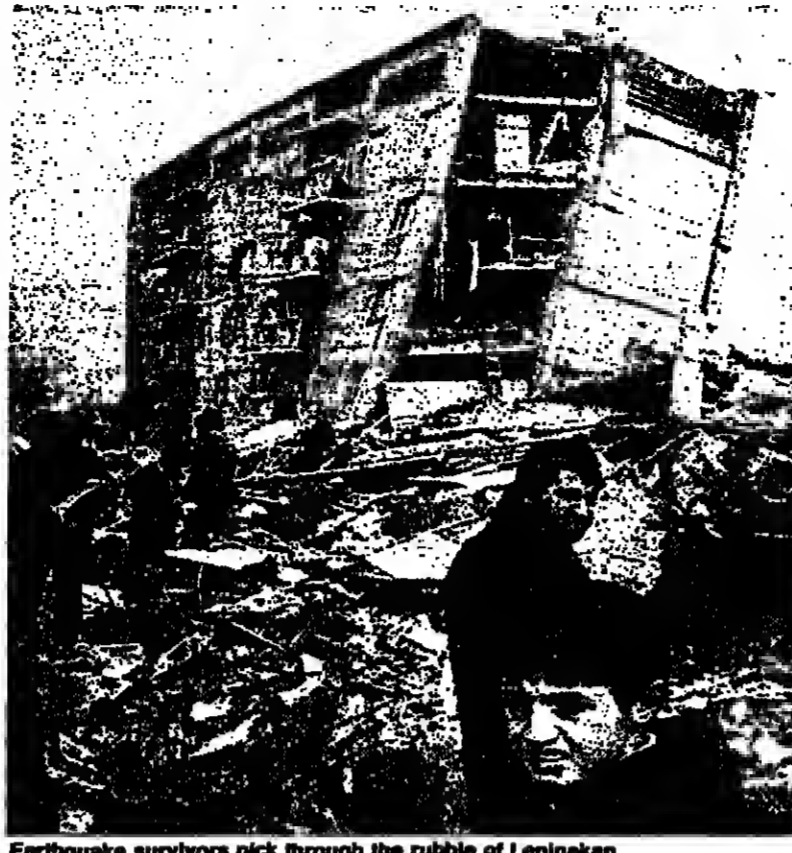
Earthquake survivors pick through the rubble of Leninakan
